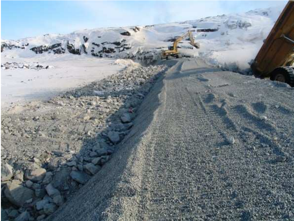
Photo 9 : Progress filling key trench.
