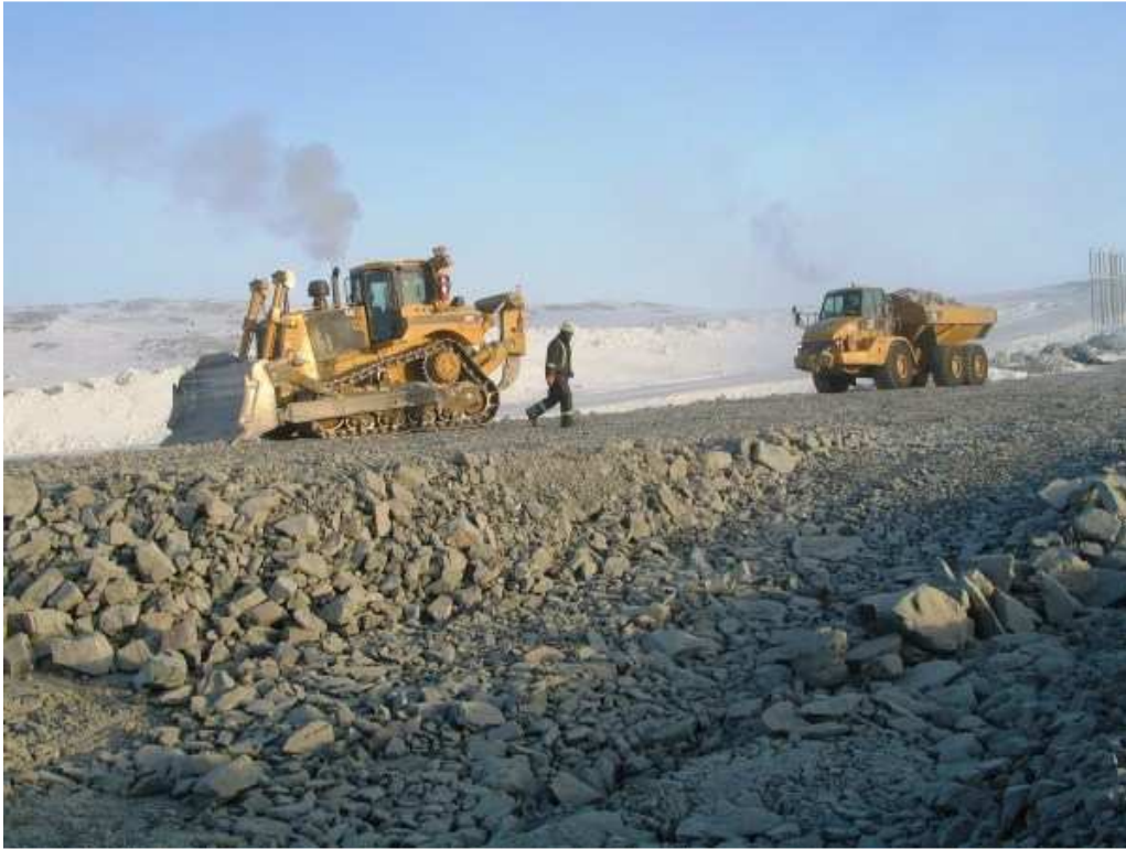
Photo 9: ROQ placement, downstream. ROQ is good quality.
