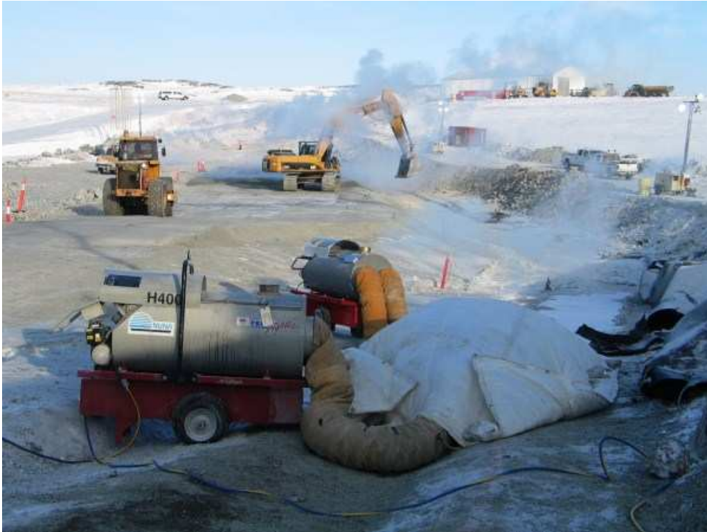
Photo 7: Frost fighters at the SE corner thawing ice over GCL.
