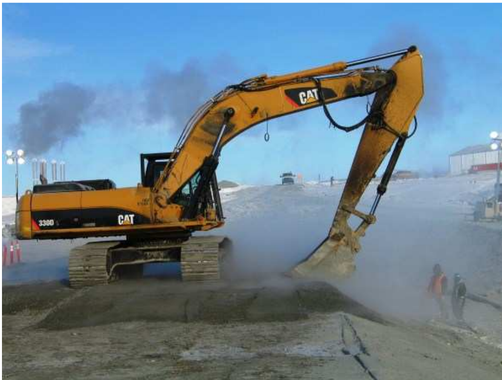
Photo 8: Placing FCM. Labourers to the right shape edges to achieve 2.5:1 slopes
