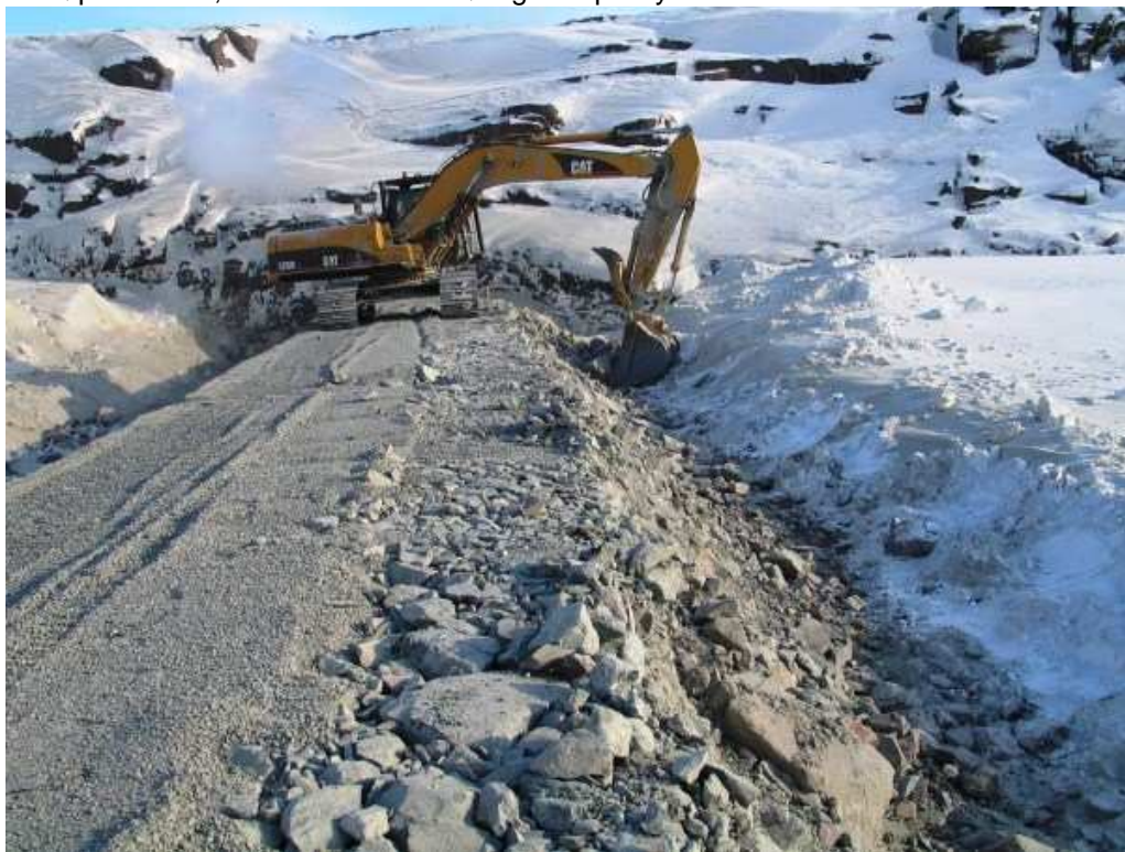
Photo 8: Reshaping the North Diversion Berm
